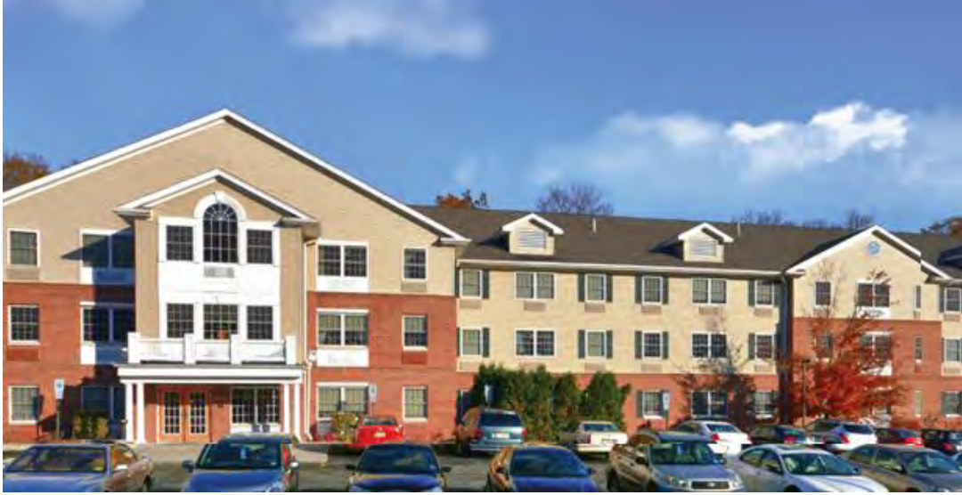
A $900,000 CIP advance helped provide construction funding for Spruce Senior Housing in Dover, New Jersey. The three-story, 90-unit senior housing complex offers its residents a full suite of amenities, including health screenings, landscaped recreation areas and a community garden, as well as access to local retail and commercial districts. This project helped revitalize the neighborhood and increased the availability of affordable housing for seniors in Morris County. (Source: The New York Bank)
